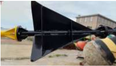
Figure 5 Topmark bolted and welded connections to be inspected
