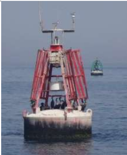
Figure 10 Bird fouling and marine growth should be cleaned
