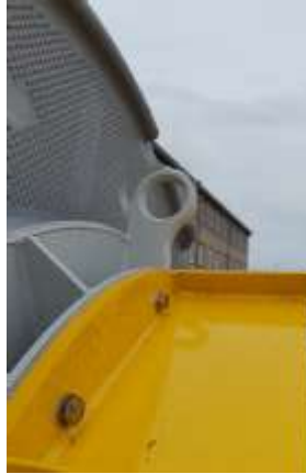
Figure 8 Topmark fasteners, welding and lifting eyes must be inspected
