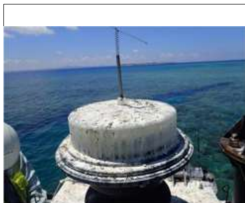
Figure 25 Bird guano fouling of lantern
